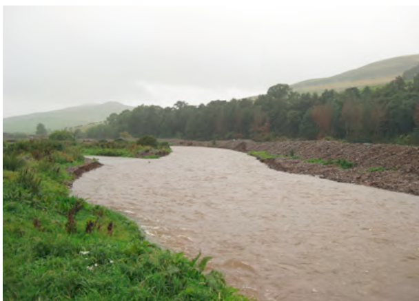
Figure 26: Bowmont Water channel dredged 05 August 2009 approx 1m below natural bed level.
